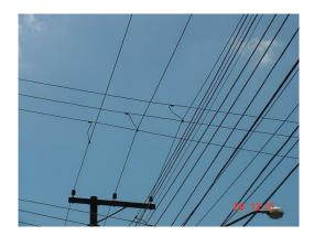
Figure 8 - Flay-tap with insufficient phase separation
